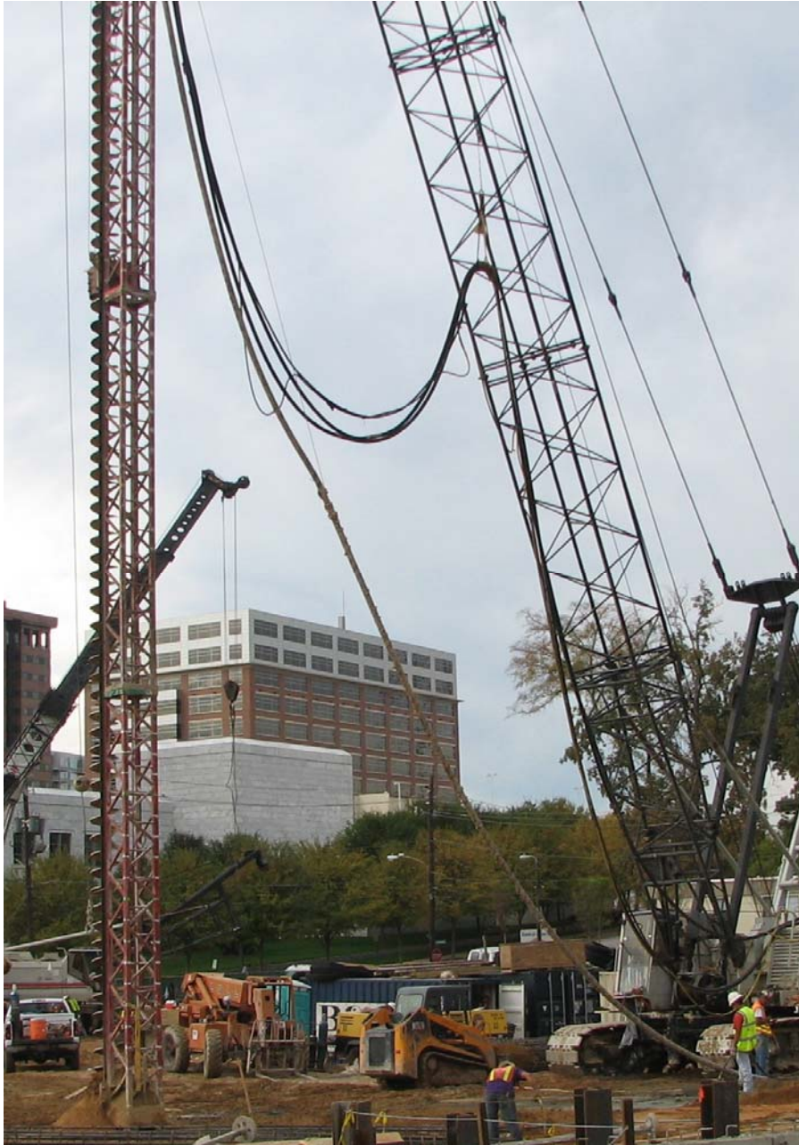
Figure 3: ACIP Installation
