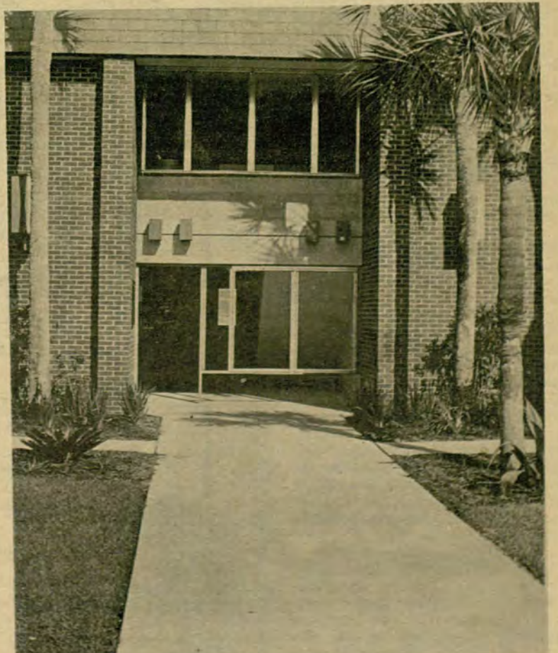
WORK on the new glass doors for the girls' dorms was well underway this week.
