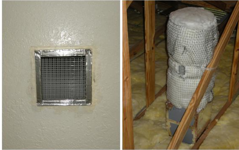
Figure 8. Ceiling penetration for planned horizontal plane leakage (left); attic view of hole that diffuses airflow (right)
