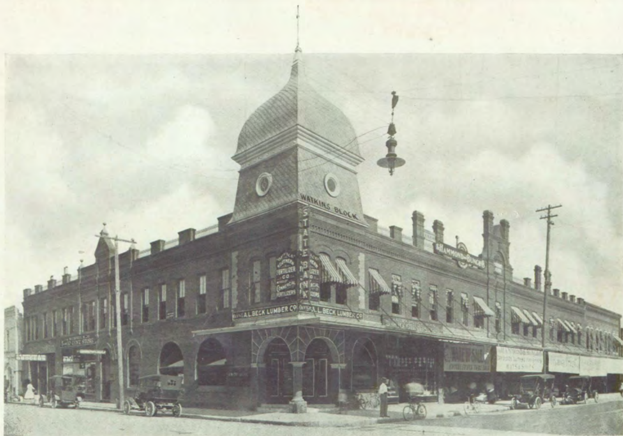
STATE BANK OF ORLANDO, CORNER ORANGE AND PINE STREETS
