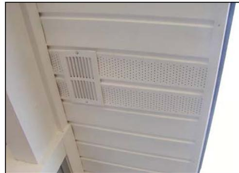
**Figure 1:** At a minimum, outside air intake register mounted in vented vinyl soffit with outside air duct positioned in soffit above. Note that a filter-back return register is preferred whereas this is a fixed register.
