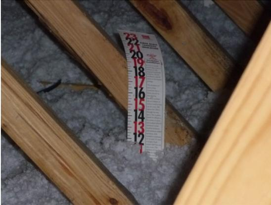
Figure 4-15. Blown insulation in attic is about 11"-12" in most areas which is about R-38.
