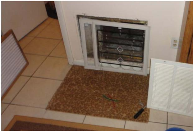
Figure 4-31. An airflow measuring plate sensor that measured air conditioner airflow is seen at the return intake. This was placed at the air handler inside the filter access slot when possible.
