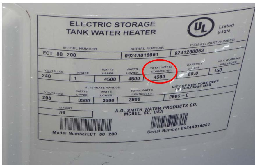
Figure 4-8. Water Heater Nameplate. This nameplate states that the total device wattage is 4,500 watts.
