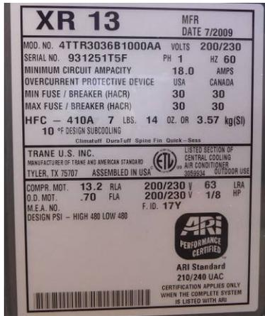
Figure 4-23. Photo of condensing unit tag. With model number listed at top of this 35.0 kbtu cooling system.
