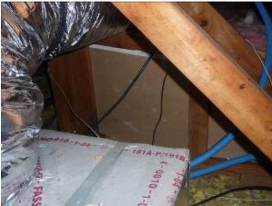
Figure 4-17. Photo shows an area of kneewall missing insulation in an old code home (H59).
