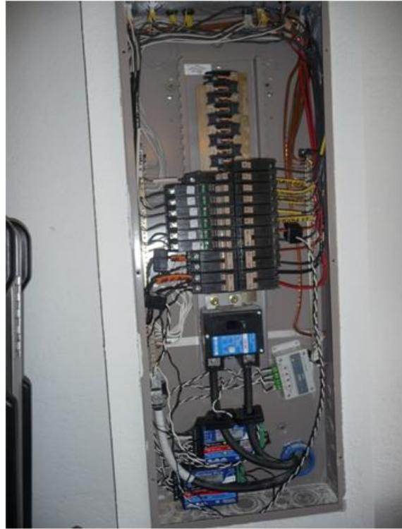
Figure 4-2. Wattnode power meters and Hobo data logger energy monitoring system after being installed in an electric panel by a licensed electrician.
