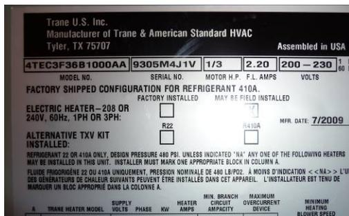
Figure 4-24. Photo of air handler unit tag with model number shown at the top. Below this tag was information indicating this system had 9.6kW of electric strip heat.
