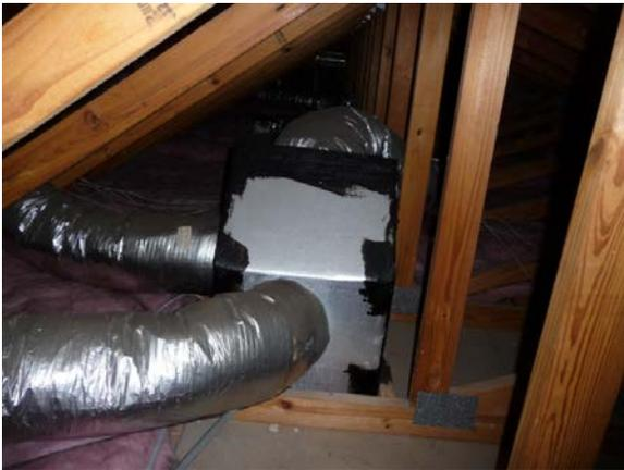
Figure 4-21. Many old code home had R-6.0 insulated ducts in attics and evidence of duct mastic applied at joints and connections such as this one with black mastic.
