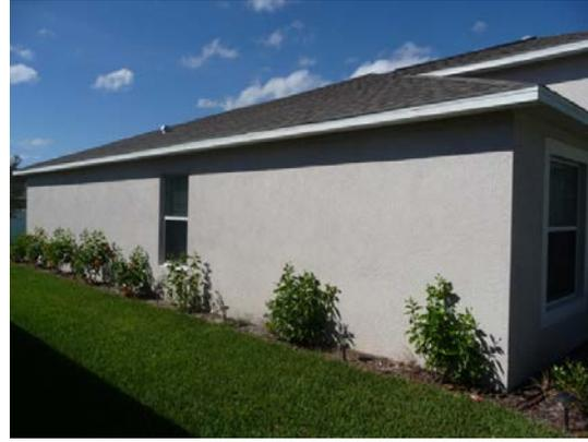
Figure 4-13. New code home (45) with little shading, but less glass area on exposed east and west sides.
