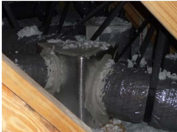
Figure 4-22. Duct inspection shows mastic and proper mechanical support was used on this new code system.
