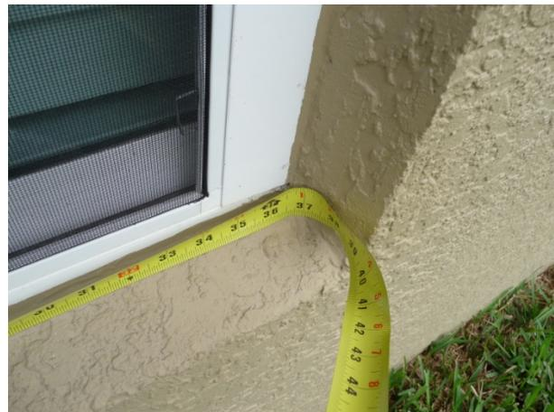
Figure 4-11. Window width measurement shown here. The type of window, height, orientation and shading related factors are also measured for every window and wall.
