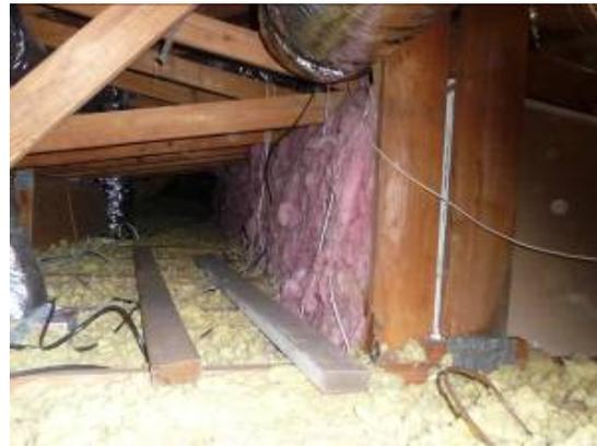
Figure 4-18. This is same house in photo at left showing kneewall insulation in decent condition around the corner from the un-insulated kneewall (H59).
