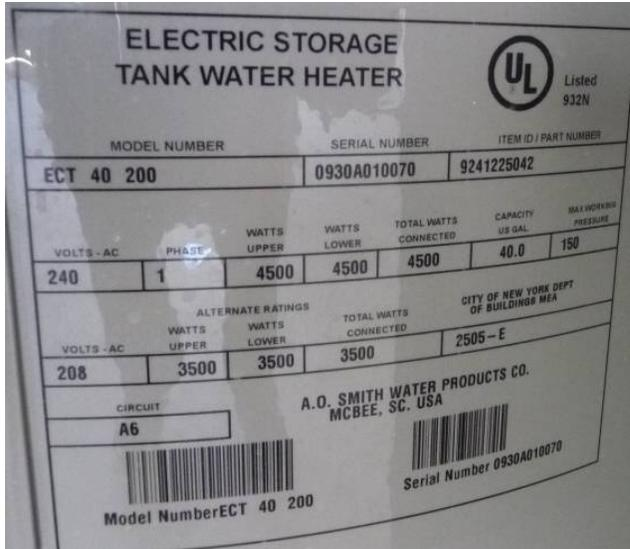
Figure 4-26. Photo taken of the 40 gallon electric storage domestic hot water heater nameplate. The model number and manufacturer are looked up using the AHRI rating directory to determine the efficiency. The rating certificate is shown below.
