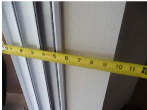
Figure 4-14 Exterior wall thickness measurement of an 8 inch masonry block wall.
