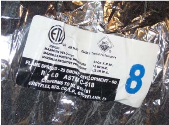
Figure 4-19. Tag on flex duct located in attic indicates R-6.0 insulation.
