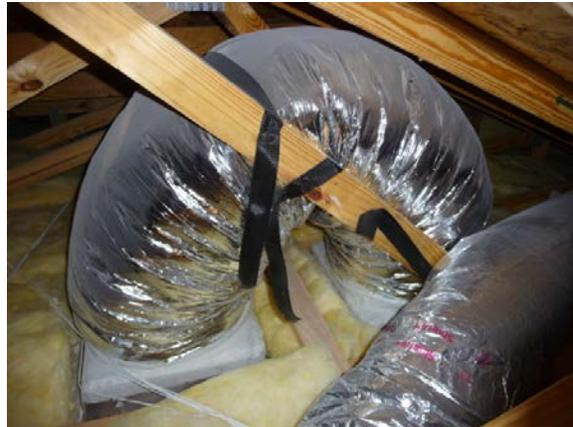
Figure 4-20. Flex duct in attic used as return air transfer (jump duct) from bedroom to central space. Mastic was used to seal connections.
