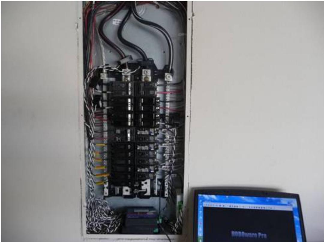
Figure 4-4. Laptop connected to installed Onset data logger is used to set up configurations and verify proper meter and logger operation.
