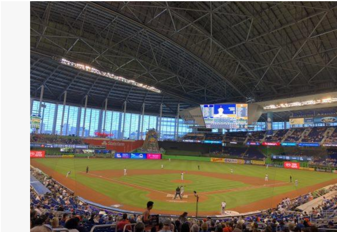
Marlins Park with its retractable roof, home of the Miami Marlins.(Photo by Fernando I. Rivera)
