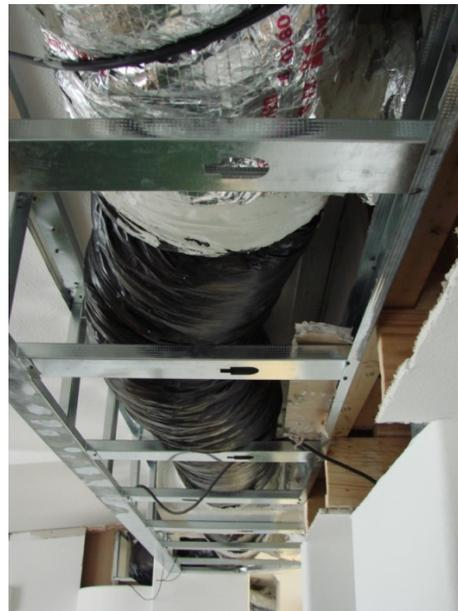
**Figure 6 MHLab soffit duct (supply side).**
