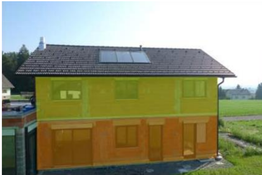
Figure 14: Construction Site Monitoring
