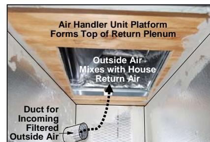
Return plenum with ventilation duct.
