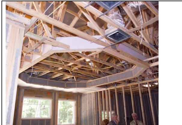
Figure 3 Solid blocking at tray ceiling framing (GWR).
