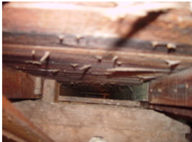
Figure 4 - Balloon wall cavity as viewed from attic
