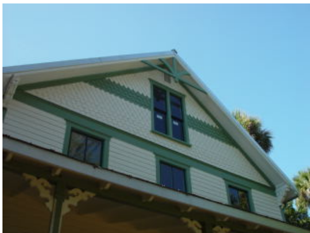
Figure 1 - Attic Window on Gable End
