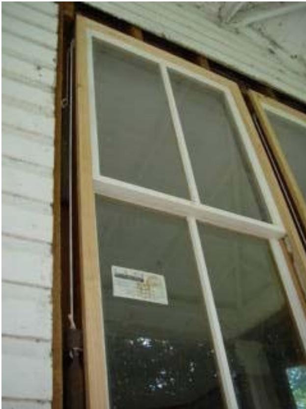
Figure 7 - Replica window with weight and pulley
