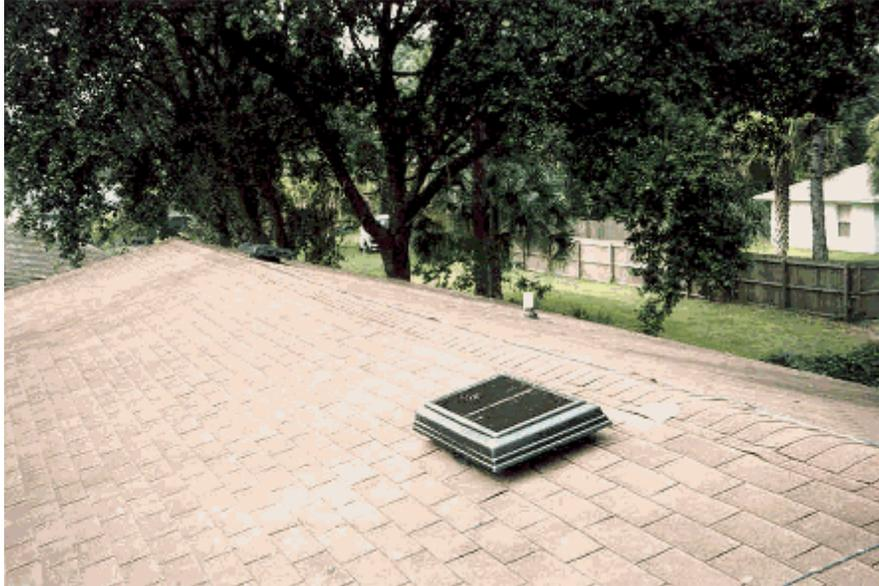
**Figure 2.** Photo of PV ventilators.
