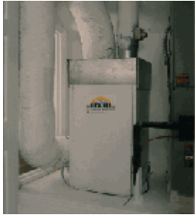
Air Handler in Conditioned Space
