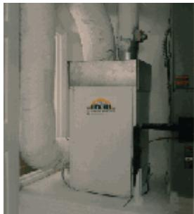
A high efficiency dehumidifier ([Figure 23](#)), provides excellent indoor air quality. This device ventilates and dehumidifies the home. This aids in the prevention of dust mite infestations, as well as inhibiting mold, mildew, and bacteria growth. The air filter is a 7" thick, high efficiency filter ([Figure 24](#)) which removes airborne particles down to one micron in size. It needs to be changed only once or twice each year. The result is a home full of clean, dry, fresh air.
