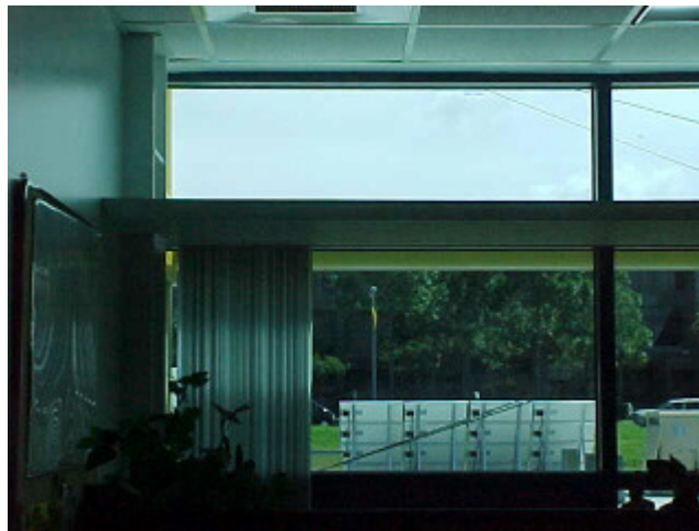
Lightshelves in the South facing windows at FSEC
