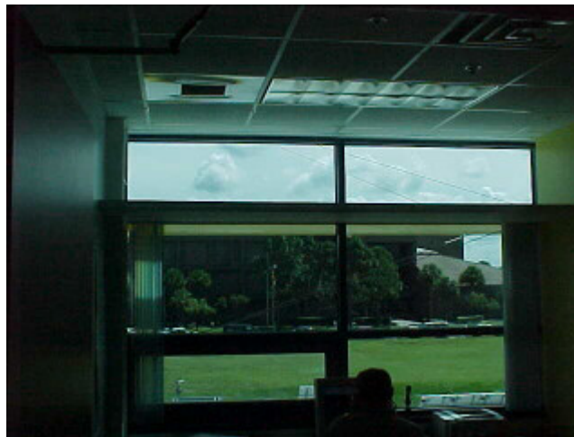
Figure 6. Interior of an office where daylight dimming and window management strategies were studied. The office has south-facing windows with a light shelf.
