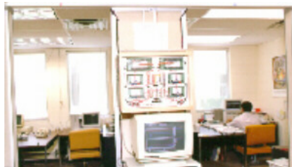
Figure 4. Lighting Flexible Test Facility (LFTF) configuration
