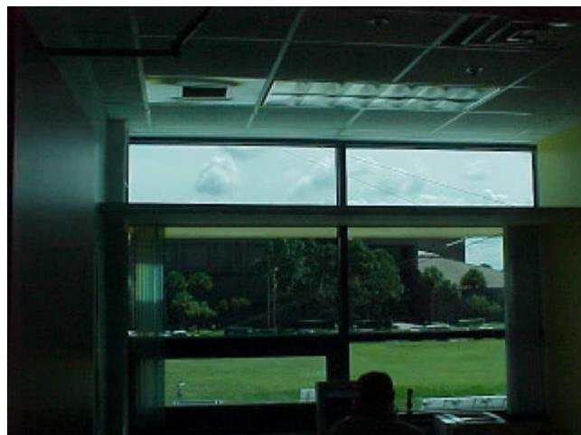
**Figure 6.** Interior of an office where daylight dimming and window management strategies were studied. The office has south-facing windows with a light shelf.
