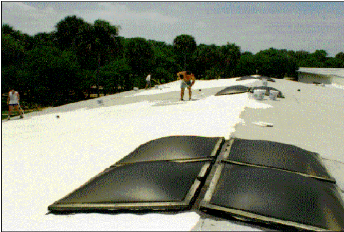
Figure 12. First of three coats of white acrylic elastomeric is applied to school roof on May 9, 1995.
