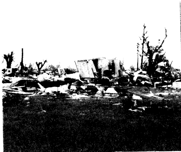
Figure 2. Illustration of Damage.
