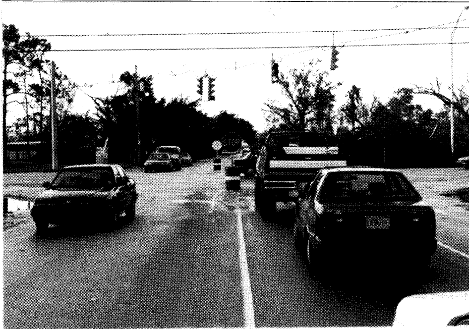
Figure 7. Partially Repaired Traffic Lights that are Difficult to Understand.
