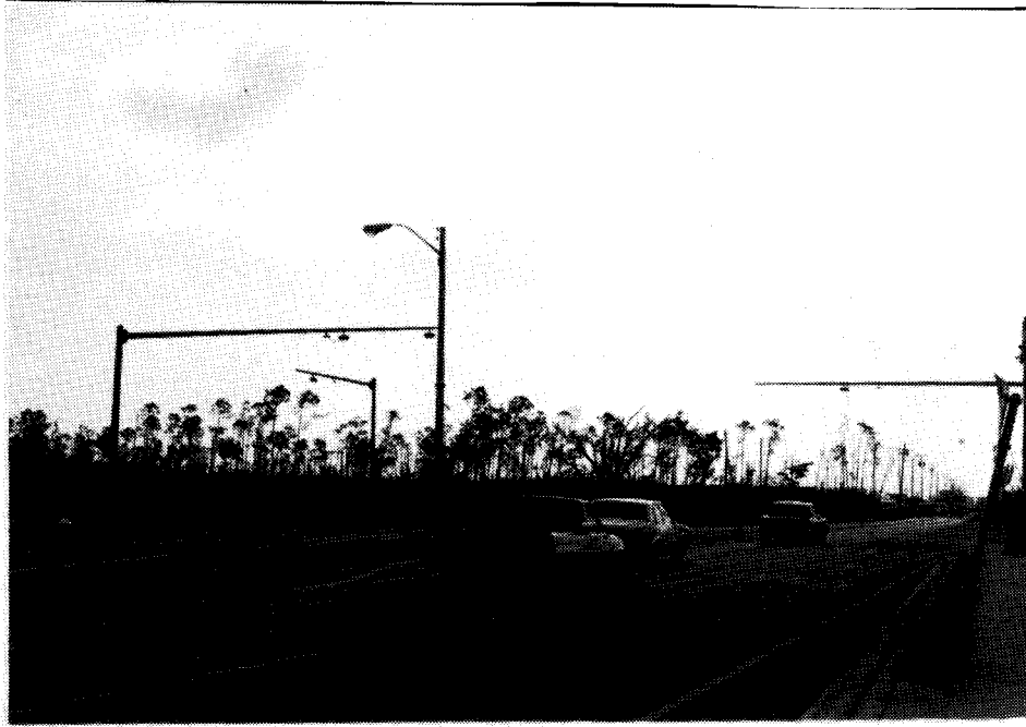
Figure 4. The Poles are Standing, but the Signals are Missing at an Intersection in Miami.
