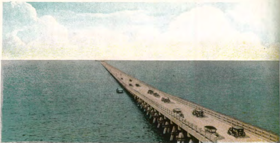
GANDY BRIDGE, LONGEST AUTOMOBILE TOLL BRIDGE IN WORLD CONNECTING ST. PETERSBURG AND TAMPA, FLA., 6 MILES LONG AND CROSSING TAMPA BAY.
