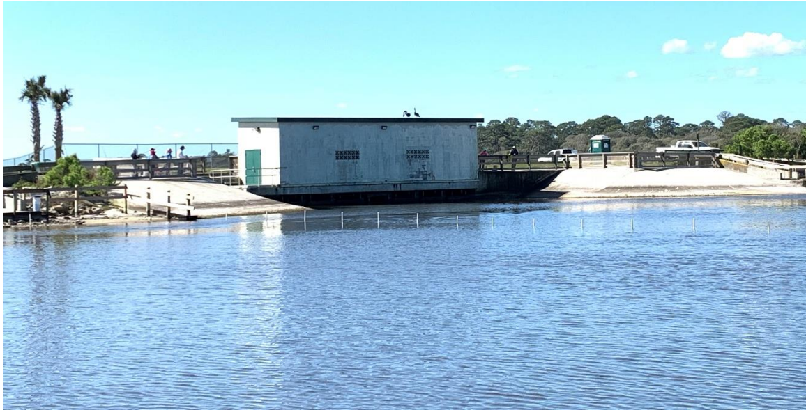
Figure 1- Guana River Dam
