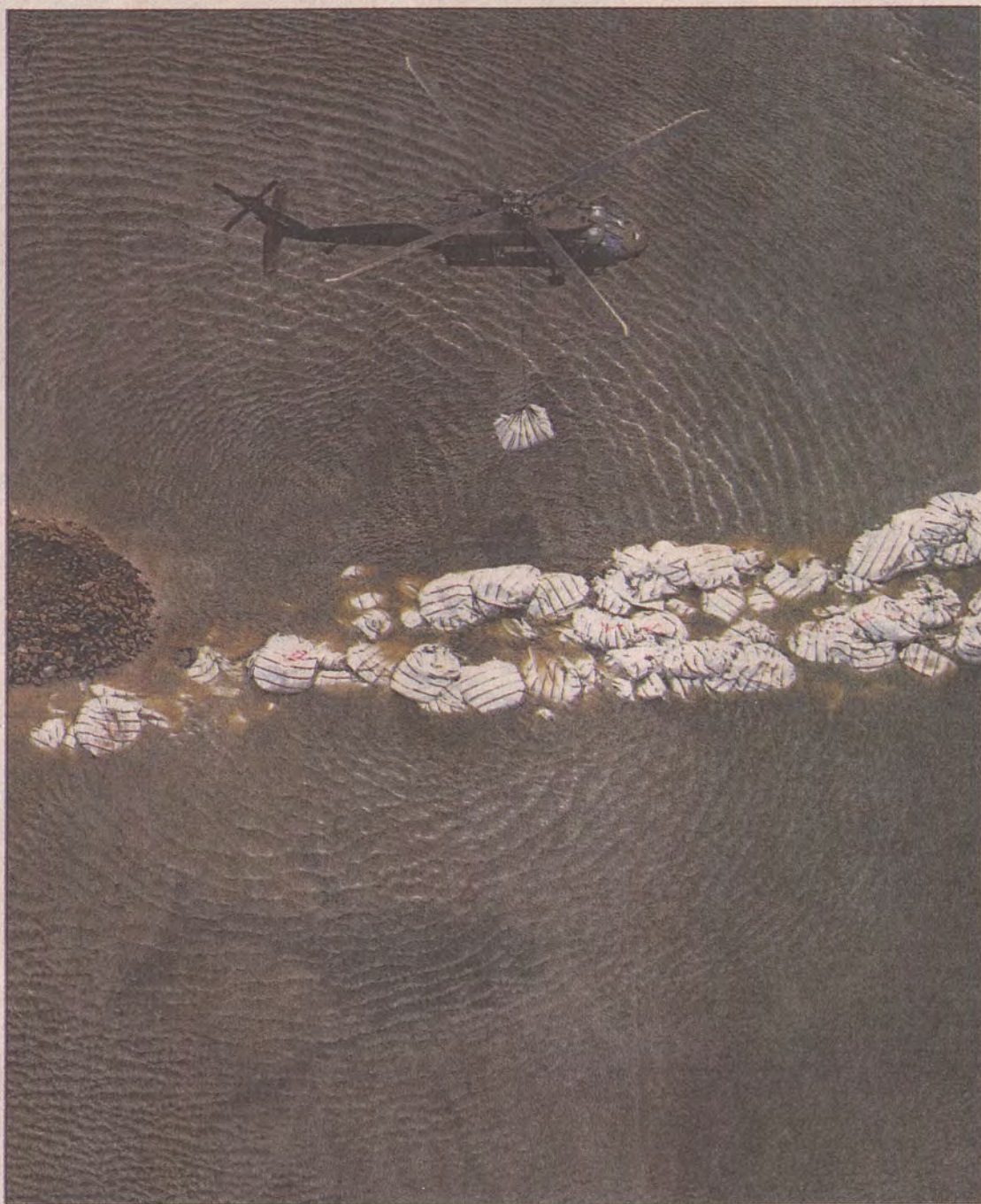
A military helicopter drops a sandbag to repair the 17th Street canal levee on Monday, Sept. 5, 2005, in New Orleans. U.S. District Judge Standwood Duval threw out a key class-action lawsuit Wednesday against the U.S. Army Corps of Engineers over the failure of a wall on the canal.
