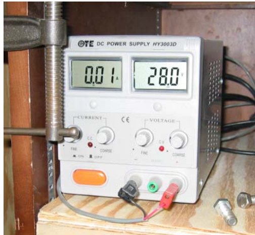
Figure 31: Pressure Transducer Power Supply
