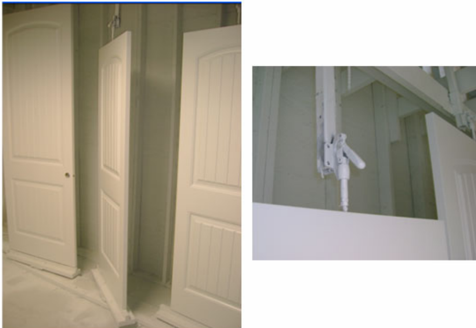
Figure 27- Door Clamp System
