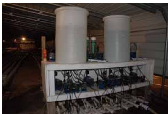
Figure 36 Inhibitor tanks and feed pumps
