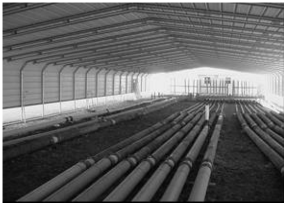
Figure 10 Pilot distribution systems
