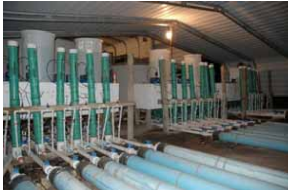
Figure 8 Influent standpipes
