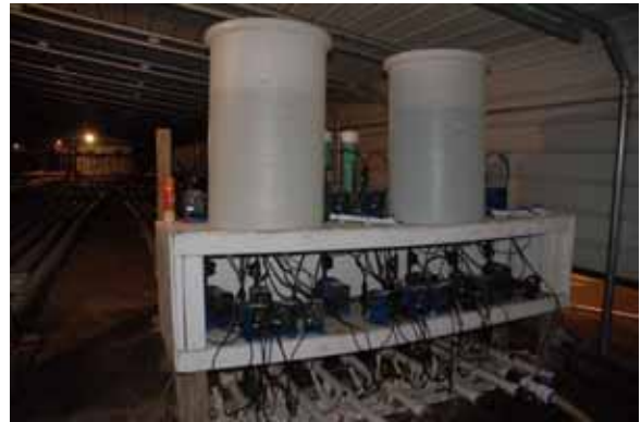
Figure 9 Inhibitor tanks and feed pumps
