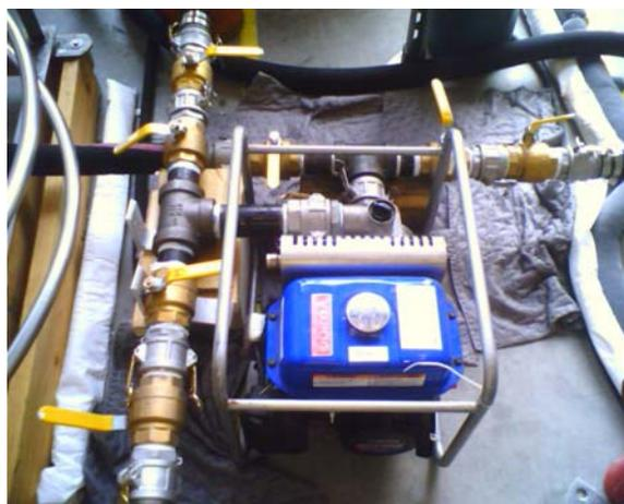
**Figure 9. Yamaha Pump, 123cc, 4-stroke gasoline driven**
