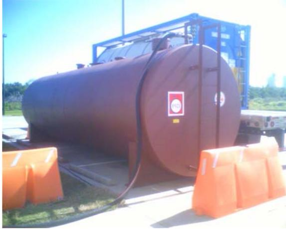
**Figure 11. Double-walled 10,000gal isotank for Petroleum Storage**
