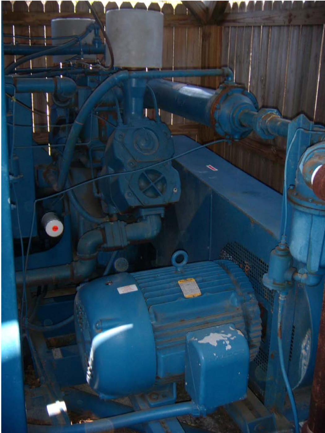
Figure A.2: Quincy Three-Piston, Two-Stage Air Compressor, Maximum Output of 0.01 kg/s at 250 psi
