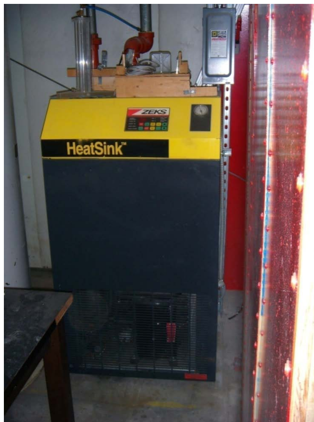
Figure A.4: Condenser and Reheater
