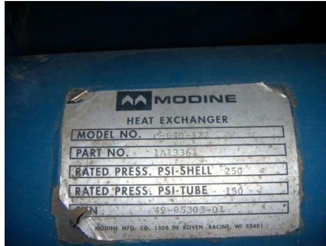
Figure A.3: Modine Heat Exchanger, Directly out of Compressor
