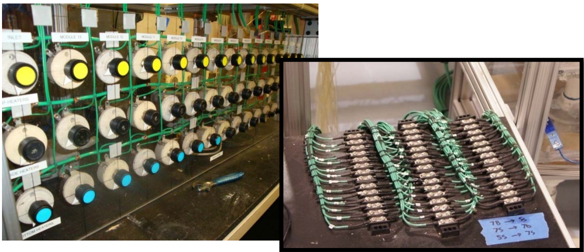
Figure 2.5: Photo of Heat Supply System
