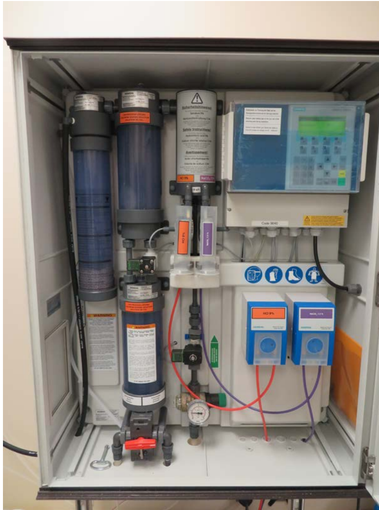
Figure 4.2 Siemens AC-10 chlorine dioxide generator
